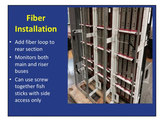
The fiber loop was installed in the middle of the rear compartment above and below structure braces. To avoid crimping or breaking the fiber loop, common PEX bend supports were installed where bends were made in the loop. Due to the available space, the use of screw together fish sticks can reach from end to end of large lineups by using the brackets for support. This allows side access to install the fiber loop.
