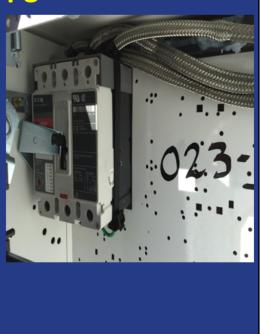
Proper torqueing of MCCB terminals (stop ejection of lead wires under fault conditions) Shielded line side jumpers to ground (stops fault propagation between phases or if lead wire is ejected under fault conditions and eliminate shock hazard)
