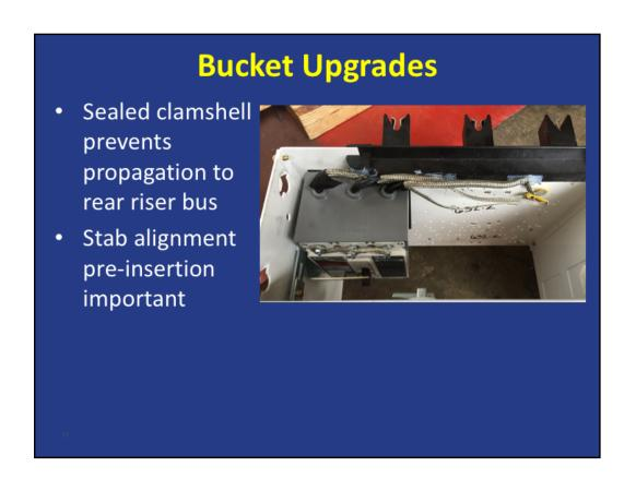
We did find several instances where stab alignment caused issues under fault conditions. Improper insertion can break the clamshell support or deform one side of the stab. We have also witnessed the stab assembly missing the riser bus completely only contacting the outside of the stab – making it electrically conductive but totally ineffective under fault conditions leading to bus compartment failure.
