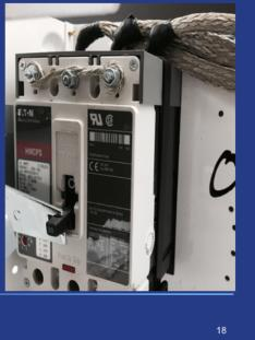
Lugs on line side of breaker were drilled and tapped to accept 8-32 screws to provide access for wrapping fine strand #10 SIS bare wire to short-circuit terminals for test.
