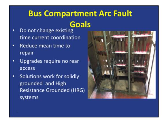
After completing the bucket modifications, we felt that we could isolate any type of fault inside the bucket to remain inside the bucket. The sealed clamshell prevented a bucket fault from propagating to the riser bus.
