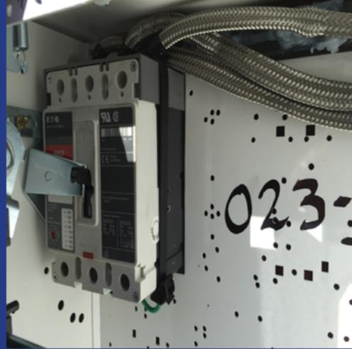
Proper torqueing of MCCB terminals (stop ejection of lead wires under fault conditions)
