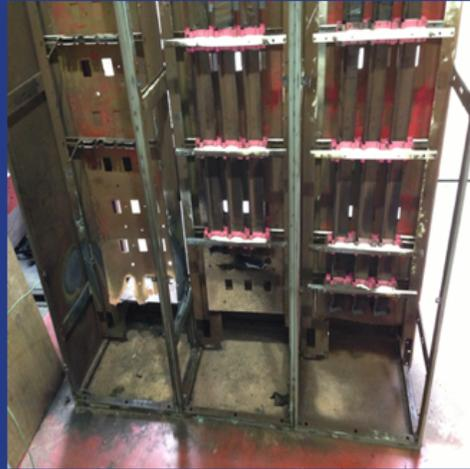
After completing the bucket modifications, we felt that we could isolate any type of fault inside the bucket to remain inside the bucket. The sealed clamshell prevented a bucket fault from propagating to the riser bus.
