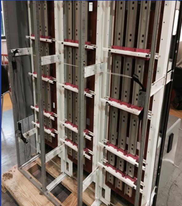
The fiber loop was installed in the middle of the rear compartment above and below structure braces. To avoid crimping or breaking the fiber loop, common PEX bend supports were installed where bends were made in the loop. Due to the available space, the use of screw together fish sticks can reach from end to end of large lineups by using the brackets for support. This allows side access to install the fiber loop.
